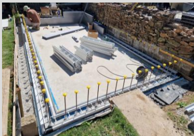
Accommodate any location of starter bars with moveable R-Ties
