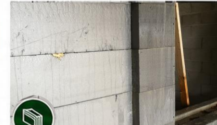
CREATE FLUSH-APPEARANCE CLADDING by altering R-Board thicknesses
