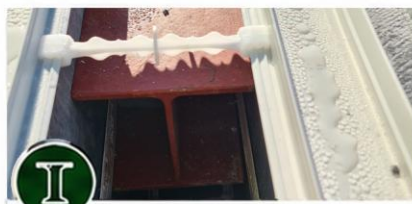
INCORPORATE I-BEAMS overcoming thermal bridging
