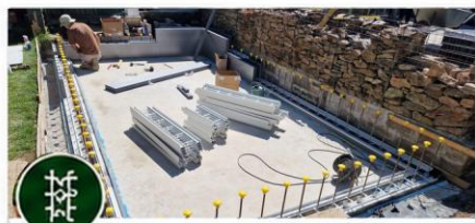
ACCOMMODATE ANY LOCATION OF STARTER BARS with movable R-Ties
