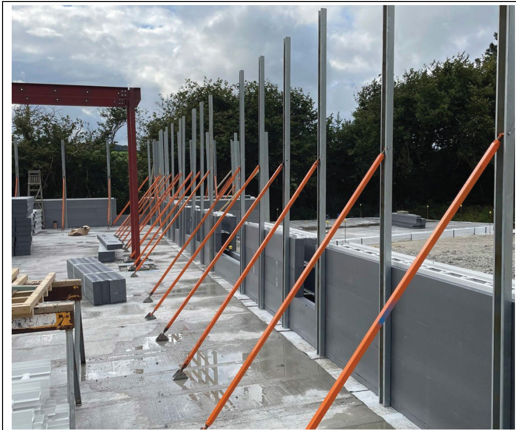
Figure 4 R-Wall Propping/support system
